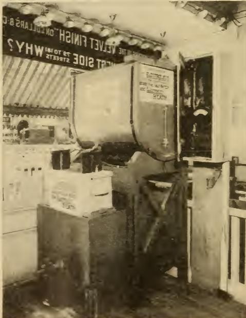
APPARATUS TO PRODUCE CHLORINE BLEACH
