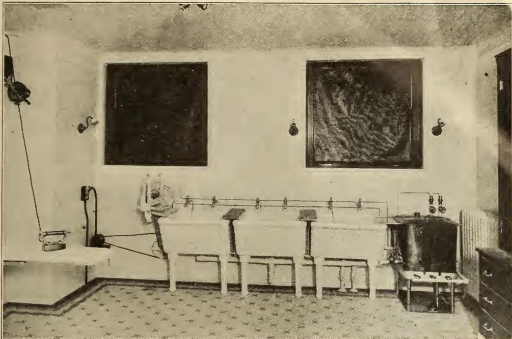
RINSING TANKS AND MOTOR DRIVEN WRINGER
