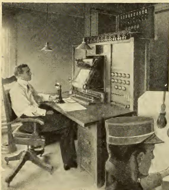
THE TRAIN DISPATCHER HAS CONTROL OF THE "STOP" AND "CLEAR" SIGNALS IN THE MOTORMAN'S CAB
