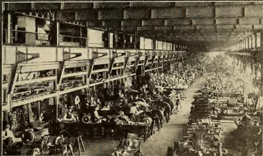
THE UPPER ONE OF THESE SHOPS IS DEVOTED ENTIRELY TO THE BUILDING OF SMALL MOTORS, IN THE LOWER ONE THE WINDING OF ARMATURES PROGRESSES—LITERALLY THOUSANDS OF THE ARMATURES ON THE BENCHES
