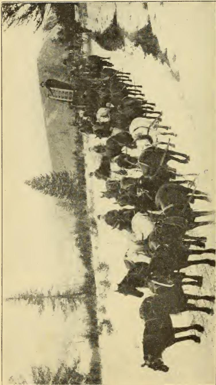
THE PROBLEM OF TRANSPORTING HEAVY ELECTRICAL APPARATUS TO PLACES WHERE NEEDED IS A HARD ONE WHEN THE PLACE OF INSTALLATION IS AWAY FROM A RAILROAD. THE ILLUSTRATION SHOWS THE FRAME CASTING OF A 700-HORSE-POWER MOTOR BEING HAULED A DISTANCE OF FOUR MILES FROM THE RAILROAD TO THE PLANT OF A BRITISH-COLUMBIA COPPER-MINING COMPANY. THE WEIGHT OF THE CASTING IS 34,000 POUNDS. NO WHEELS AVAILABLE COULD SUPPORT THE WEIGHT SO IT WAS HAULED ON RUNNERS AND AT A TIME WHEN SNOW WAS ON THE GROUND.
