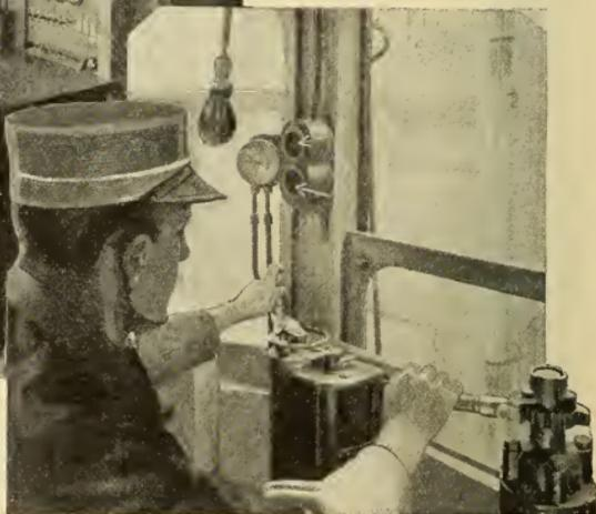
other two are termed "distant" rails. These three third rails are connected by a single wire along a pole line direct to the dispatcher's office. When a car passes them, a contact shoe attached to the side of the car truck touches a "distant" rail first. This completes the circuit from the "distant" rail through a relay or electromagnet on the car and through the truck and wheels to the track, thus putting the car relay in circuit with the dispatcher's office.
