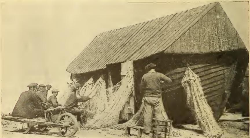
Fishermen of the Channel ports of Normandy frequently convert their fishing boats into houses by adding a roof as shown in the picture.
