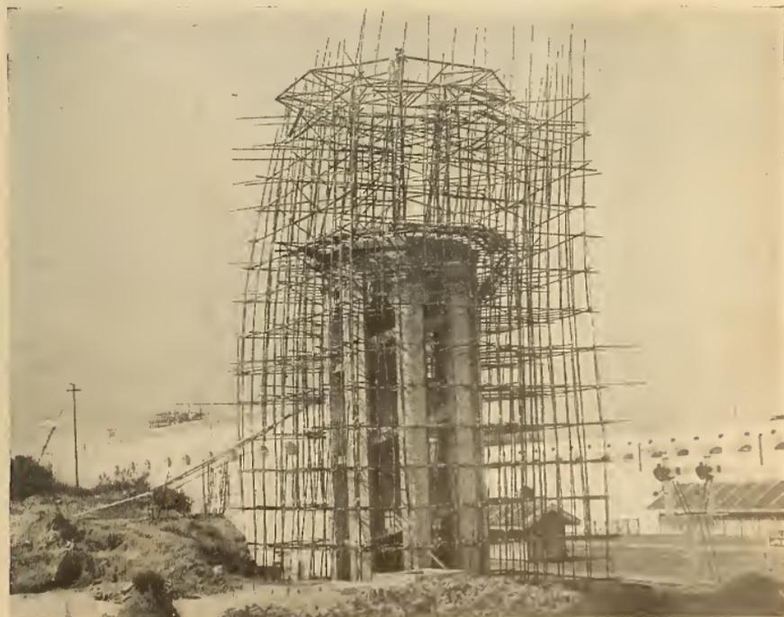
Peculiar way of building a water tower in Kuala Lumpur, Federated Malay States. A huge scaffold made of bamboo was first erected.
