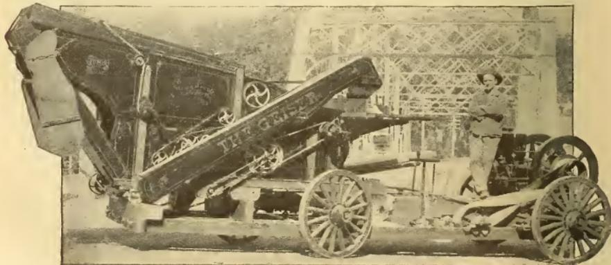
Threshing Outfit of Small Capacity but Portable and Extremely Easy to Handle
