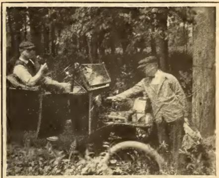
Testing a Telephone Line with an Automobile Magneto
