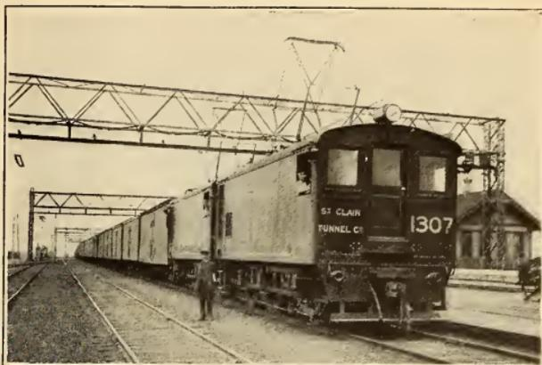
Electric Locomotive of the St. Clair Tunnel at Port Huron, Mich. It is capable of Hauling the Heaviest Freight and Passenger Trains through the Great Bore
