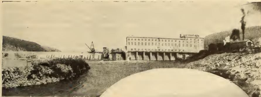
the dam is the power house, in reality part of the dam. A passage way  $2\frac{1}{2}$  by  $6\frac{1}{2}$  feet extends through the dam from end to end so one may pass from the power house to the lock. This tunnel serves also for wires to conduct current to the motors operating the lock gates.
