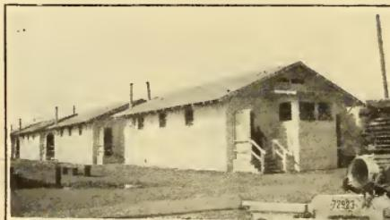
Temporary Class Rooms Erected for Los Angeles Schools, Made Necessary by Rapid Growth of Certain Districts. As Soon as Permanent Buildings Can be Erected, the Temporary Ones Are Knocked Down, and Transported by Motor to Other Localities.
