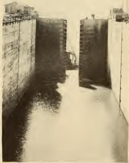
The Great \$9,000,000 Hydro-Electric Plant at Hale's Bar on the Tennessee River. A Vast Lake Was Formed by the Impounded Waters. The Locks, Permitting Navigation, have a Lift of 59 Feet, the Highest in the Western Hemisphere.
