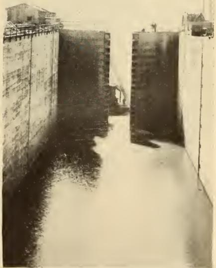
The Great \$9,000,000 Hydro-Electric Plant at Hale's Bar on the Tennessee River. A Vast Lake Was Formed by the Impounded Waters. The Locks, Permitting Navigation, have a Lift of 59 Feet, the Highest in the Western Hemisphere.
