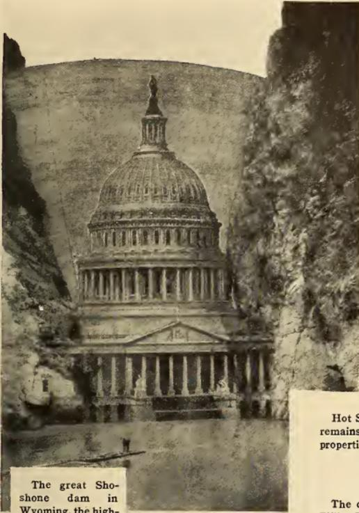
The great Shoshone dam in Wyoming, the highest in the world, is a wedge of concrete 328 feet from base to top. Were the U. S. capitol set down in this gap the tip of the dome would fall short of the dam parapet some 21 feet.
