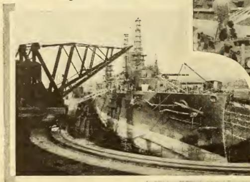
Fifty Ton Cranes Travel around the Ship on Rails
