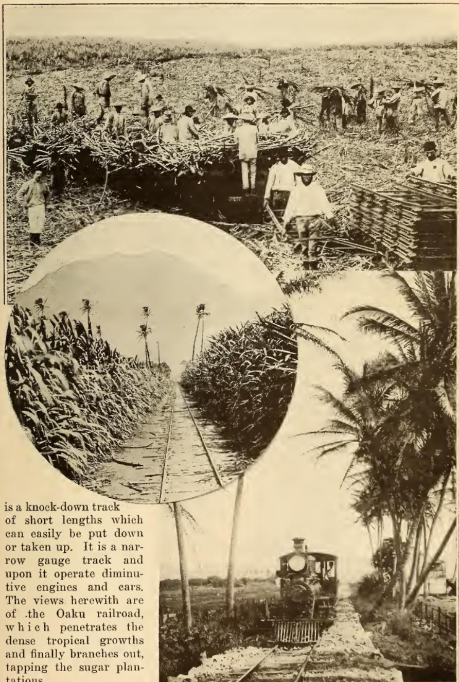
is a knock-down track of short lengths which can easily be put down or taken up. It is a narrow gauge track and upon it operate diminutive engines and cars. The views herewith are of the Oahu railroad, which penetrates the dense tropical growths and finally branches out, tapping the sugar plantations.
