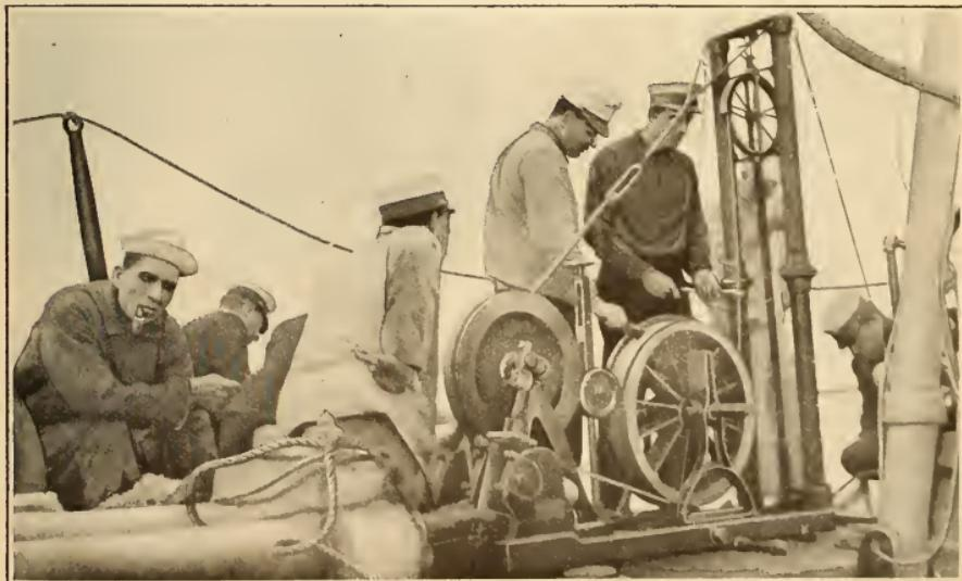
Instrument Used on United States Naval Steamship to Determine Depth of Water at a Particular Point
