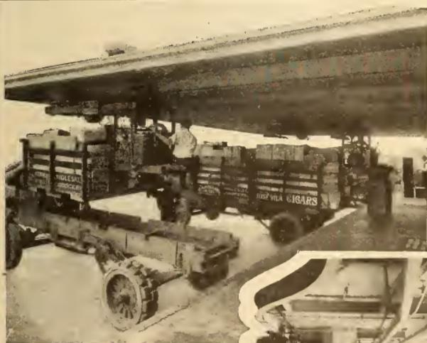
The Loading of a Truck by the Telepher System Using Removable Truck Bodies
