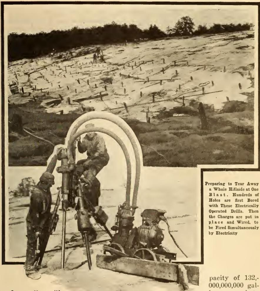
Preparing to Tear Away a Whole Hillside at One Blast. Hundreds of Holes are first Bored with These Electrically Operated Drills. Then the Charges are put in place and Wired, to be Fired Simultaneously by Electricity
