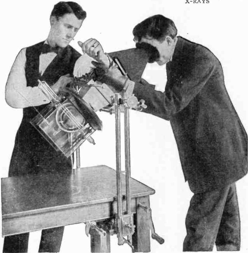
FIG. 2. MAKING A FLUOROSCOPE EXAMINATION WITH X-RAYS
