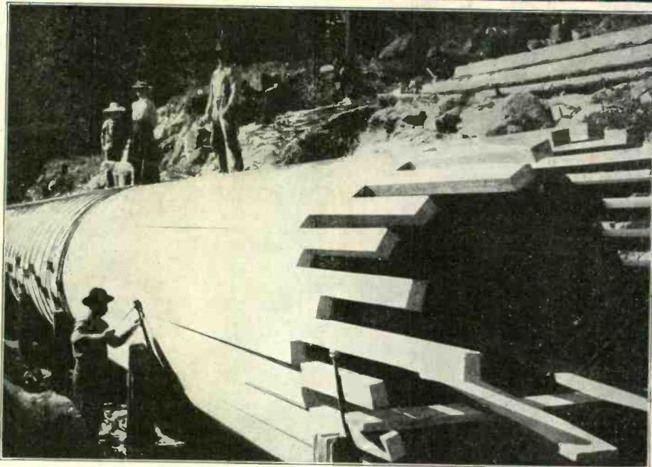
WATER THROUGH THIS PIPE LINE OF WOOD IS TO DRIVE ELECTRIC GENERATORS
