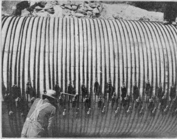
PIPE LINE OF WOOD STRENGTHENED WITH BANDS OF STEEL
