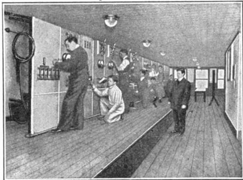
STUDENTS ENGAGED IN OPERATING A. C. AND D. C. SWITCHBOARD INSTALLATION
