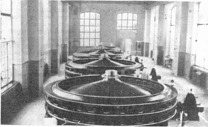
DYNAMOS IN A SWISS POWER PLANT, DRIVEN BY WATER TURBINES
