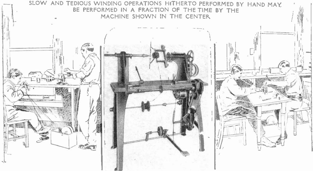
winding a drum armature and a ring armature. Yet so flexible is the machine that in a few moments it may be adjusted to do either. In addition it winds solenoid coils, transformer fields and induction coils; even more, it embodies an adjustable coil form, a very simple device which, attached to the winder, actually forms up the coils, after they are wound, to any desired shape.
