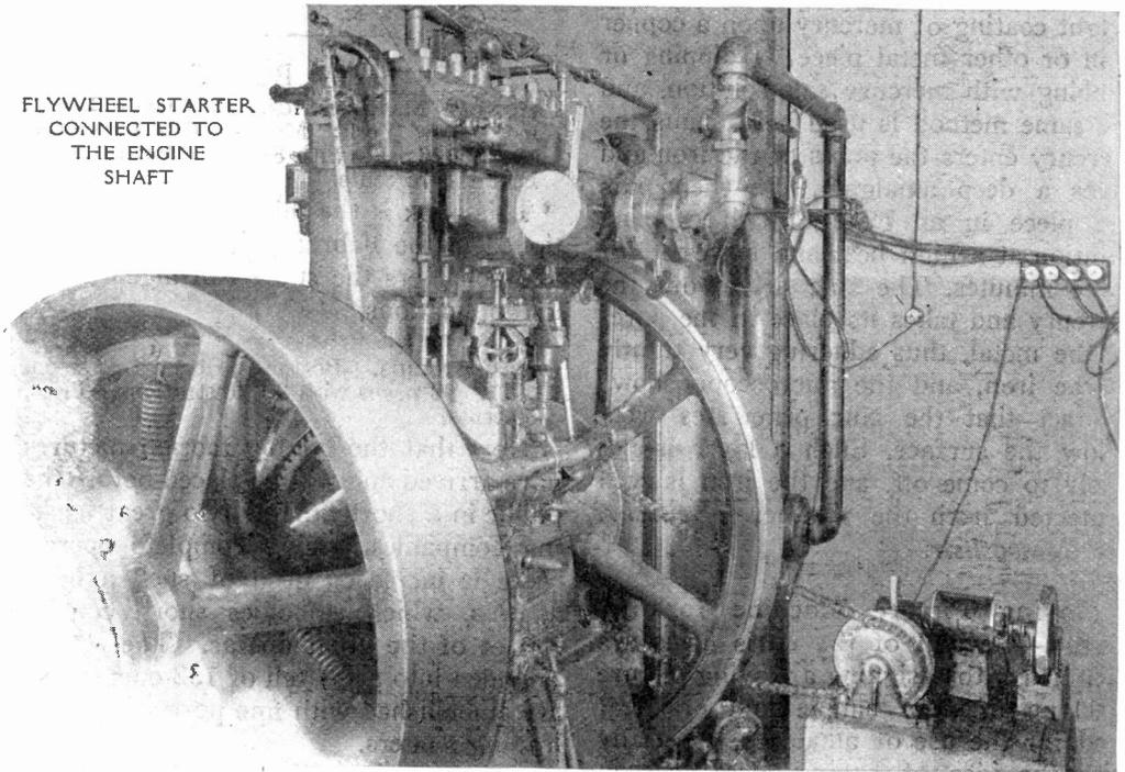
stroke of the piston before the charge can be exploded and start the engine to running of itself. This operation is most familiar in the laborious cranking of an automobile engine. In stationary engines, too large to crank by hand, the work is often done by a separate compressed air equipment, which is expensive and, if it fails to accomplish its purpose,
