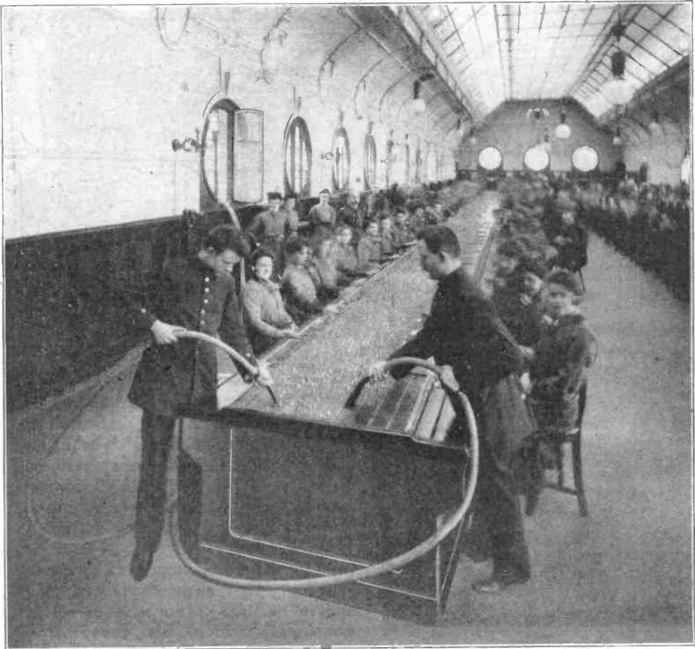
SOME OF THE TELEPHONE SWITCHBOARDS IN GERMANY ARE PLACED HORIZONTALLY AND ARE CLEANED WITH VACUUM CLEANERS
