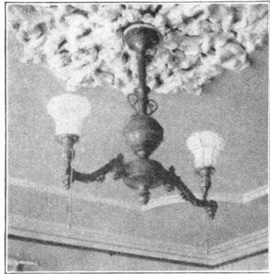
GAS FIXTURE CONVERTED TO ELECTRIC
