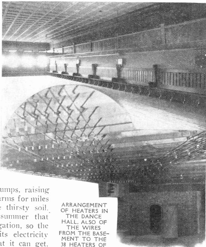
ARRANGEMENT OF HEATERS IN THE DANCE HALL, ALSO OF THE WIRES FROM THE BASEMENT TO THE 38 HEATERS OF THE BUILDING
