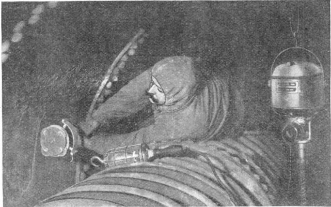
REMOVING BOILER SCALE
