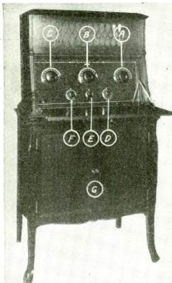
*A, B and C are the tuning dials. D, E and F are the rheostats and volume control. G is the container for the batteries.*
