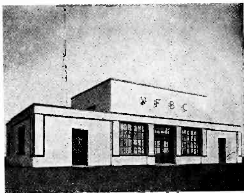
The new ultra-modern transmitter house of WFBC, Greenville, South Carolina. Also included in this house are living quarters for the engineer, a garage and workshop. It is located on the Atlanta Highway (U. S. No. 29) four miles out of Greenville.
