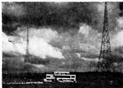
People in Switzerland should enjoy good radio reception. There are only five broadcast band stations there, but two of them are super-powered 100,000 watters. Here is the Ecomunster Sender, one of the giants. It works on 556 kcs.
