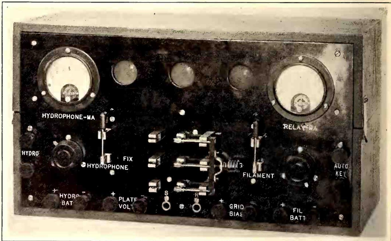
Hydrophone or under-water microphone used in new method of determining ship's position. This is submerged 60 feet under water just off shore, as at the end of the pier shown in the picture on page 11.
