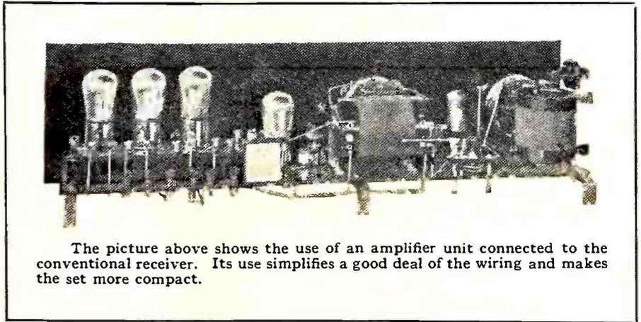
The picture above shows the use of an amplifier unit connected to the conventional receiver. Its use simplifies a good deal of the wiring and makes the set more compact.
