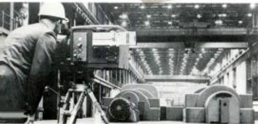
An infrared camera is used to make a thermal map of a turbine generator. The resulting thermogram (upper photo) shows temperature distribution within the generator.
