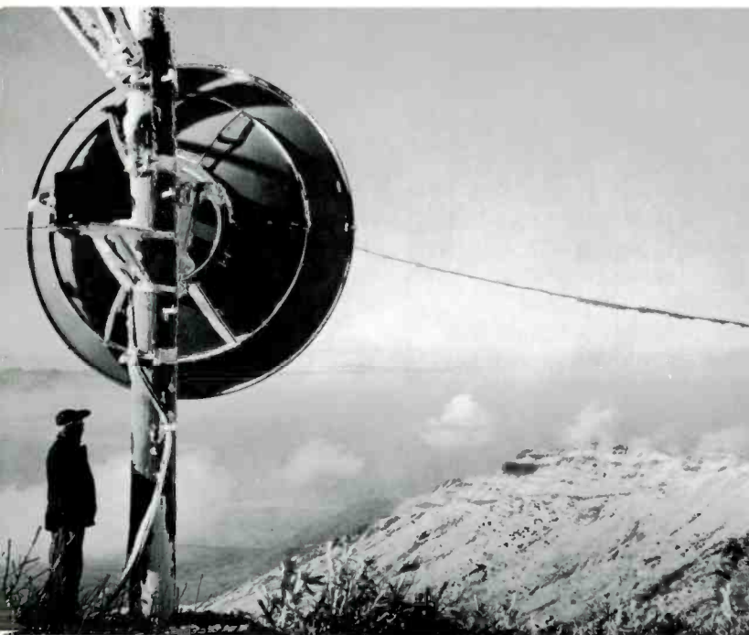
This snow-encrusted microwave antenna above the clouds in Utah beams TV programs 136 miles to a receiving station in Idaho.
