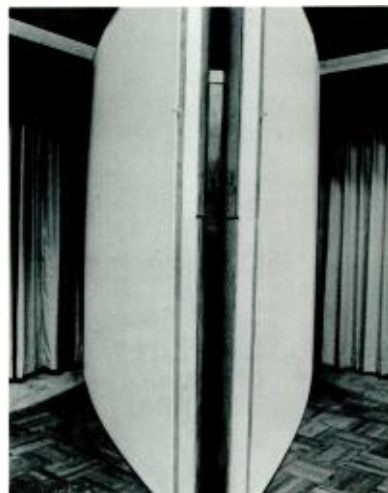
Hinged panels that can be positioned to absorb or reflect sound give two of the new RCA studios in New York a variable reverberation time.
