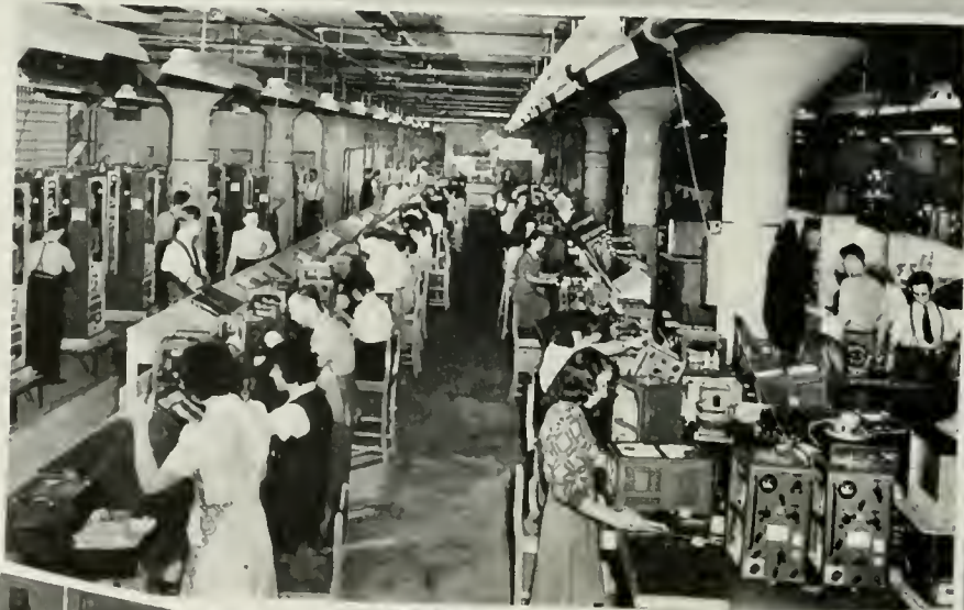
THIS LONG ASSEMBLY LINE PRODUCES THE HIGH FREQUENCY UNIT OF AIRCRAFT TRANSMITTERS.
