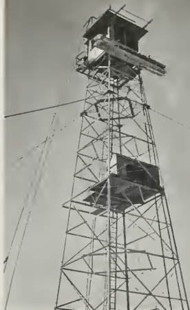
TOWERS SIMILAR TO THE ONE ABOVE SUPPORTED TELEVISION CAMERAS AND TRANSMITTERS ON BIKINI. AT RIGHT: "DRONE" PLANE CARRYING A TELEVISION CAMERA, COMES IN FOR A LANDING. OPERATOR IN FOREGROUND HAS TAKEN OVER CONTROL FROM THE "MOTHER" PLANE IN THE DISTANCE.
