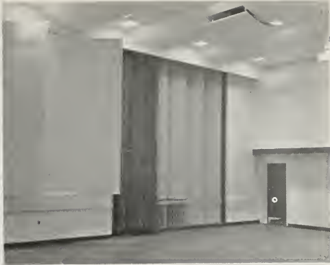
VIEWS OF NBC STUDIO 3A SHOWING UNEVEN WALL SURFACES WHICH CAN BE ADJUSTED TO CONTROL ECHOES.
