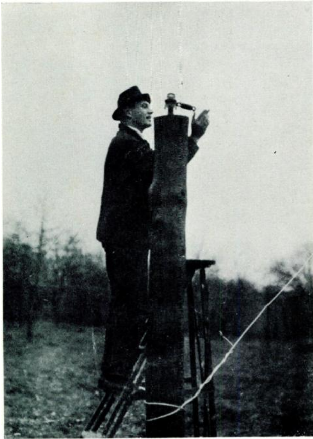
Amy inspecting the counterpoise during construction.
