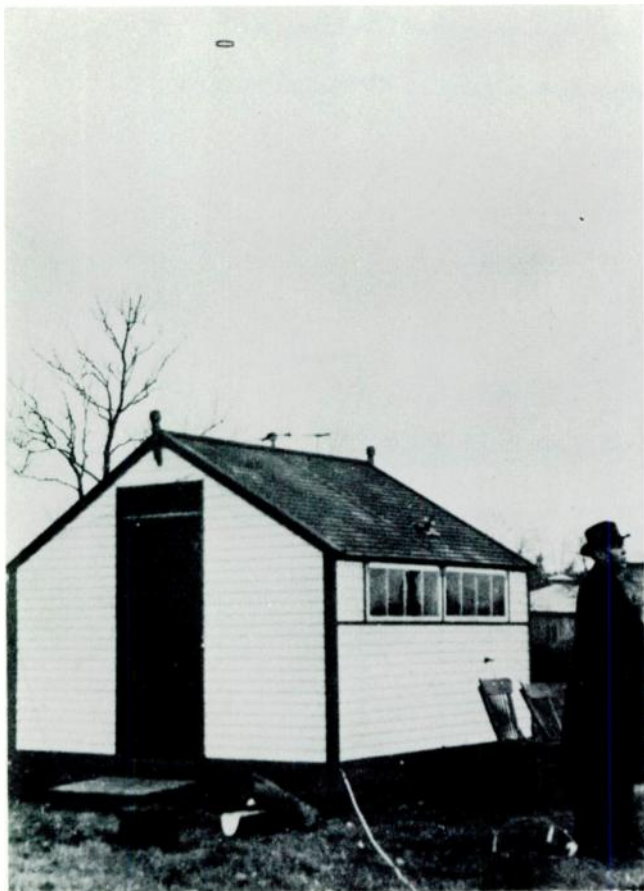
Armstrong at right, supervising construction.
