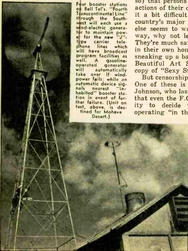
Four booster stations on Bell Tel.'s "Fourth Transcontinental Line" through the Southwest will each use a wind-electric generator to maintain power for the new "J" type carrier telephone lines which will have broadcast program facilities as well. A gasoline-operated generator will automatically take over if wind-power fails; while an automatic device signals nearest "inhabited" booster station in event of further failure. (Unit on test, above, is destined for Mohave Desert.)
