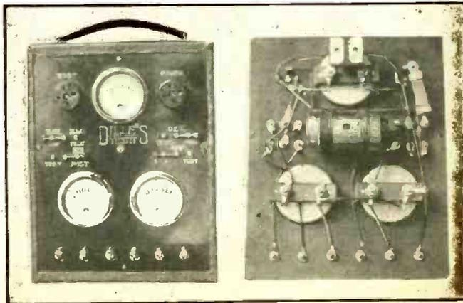
Mr. Alf. E. Dille, of Grinnell, Iowa, built this tube and set tester away back when the "X" base first came out and when most of the radio tubes were of the 200 and 201A types. This was even before the "C" batteries came into general use. Notice the old-fashion sockets, knife switches, and magnetic-vane type meters used on the front panel.
