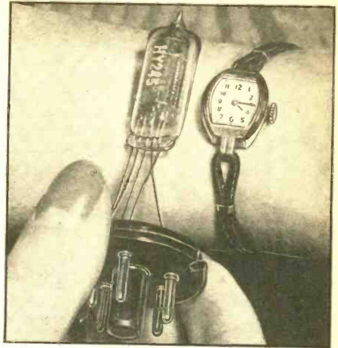
tube types are required for constructing high-gain audio amplifiers for use as hearing-aids, etc. Note that fairly wide variations in circuit constants are tolerable when these hearing-aid tubes are employed.
