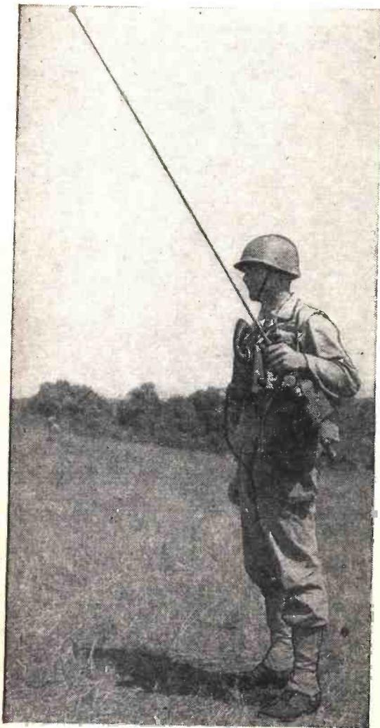
The Guidon radio as adapted for foxhole use.
