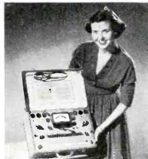
operating conditions, which takes relative tube life into account. Twelve sockets provide for testing four-, five-, six-, seven-, eight-, and nine-pin tubes; octal and lock-in miniatures; sub-miniature, acorn, and hearing-aid types; mobile and ruggedized tubes; and pilot lamps.
