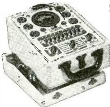
Check octals, loctals, bantam jr., peanuts, television miniatures, magic eye, hearing aids, thyratrons, the new type H.F. miniatures, etc.
