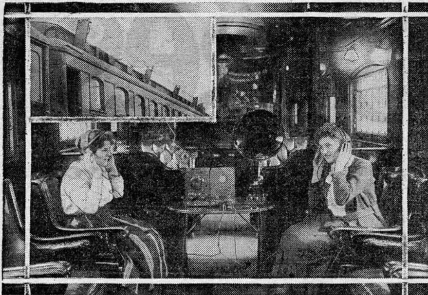
Hearing KYW, Chicago, aboard C., M. & St. P. Fast Train; insert shows antenna on roof of coach
