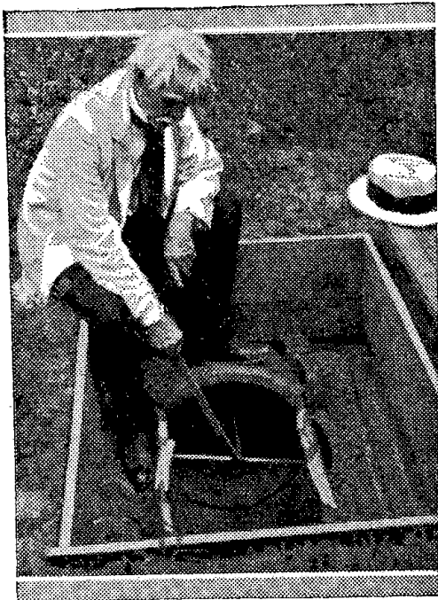
Dr. Rogers at the lead-in end of one of his static-free aeri-als. Note the hollow tile, through the center of which the underground aerial runs.
