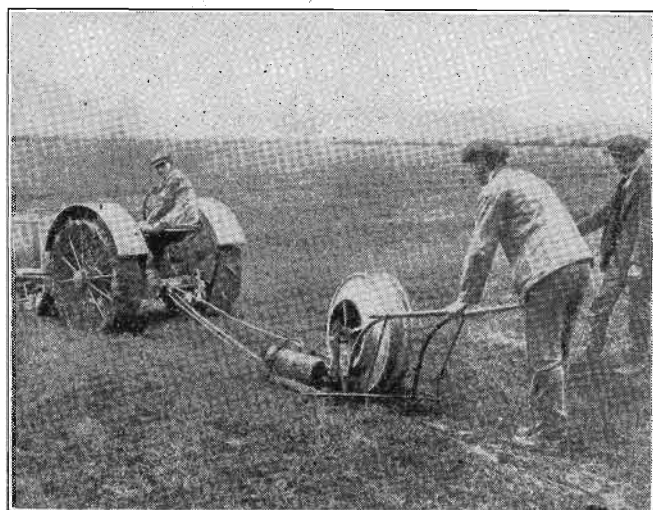
W EAF with its 50,000 watts is small potatoes compared with the new British Post Office station at Rugby, which generates 540,000 watts. Picture shows special plow that turns up a furrow just wide enough to take the wire from the drum, mounted behind.
