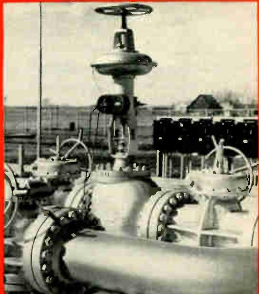
Microwave operates valves along the pipe line.
