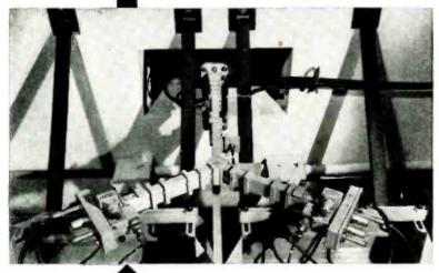
The waveguide continues upward through the roof of the station toward the antennas.
