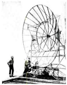
Used for reception of television signals from field pickup units, this parabolic receiving-antenna reflector is the largest in the U.S. It aperates on a 100-faot track atop Mt. Lee in Hollywood, Calif. Constructed for the Don Lee Broadcasting System, the reflector stands 16 feet high. It can be pointed at any location in the surrounding area to pick up r.f.
