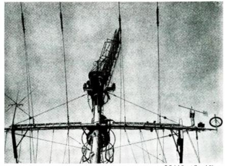
Official Coast Guard Photos Masthead of one of the ships, showing assemblage of radio and radar antennas.
