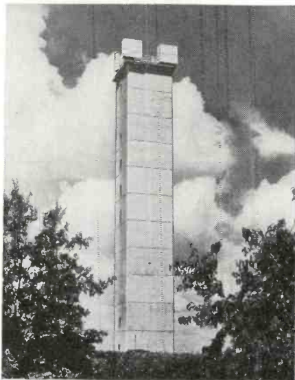
This concrete tower is one of the 34 stations between New York and Chicago.
