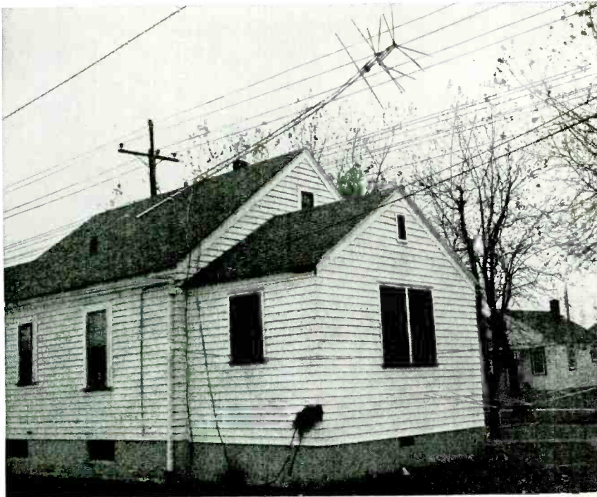
Photo A—Inadequate guying, despite its height and weight-adding rotator, caused this mast to fall across power wires, causing both injury and damage.
