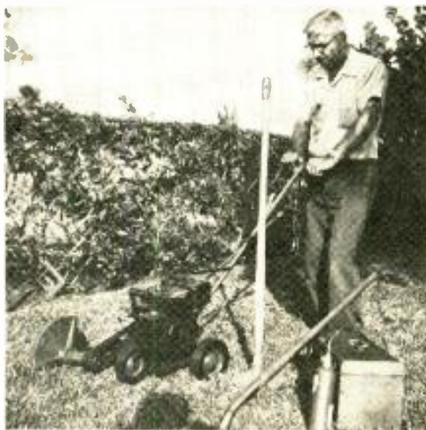
Converted lawn trimmer digs trench. Cable is inserted and ground tamped.
