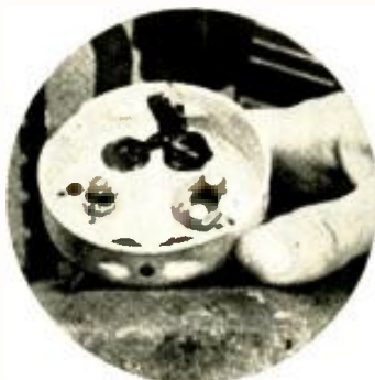
Where cable enters tapoff box the braid and insulation are rolled back to form grommet—joint then made weathertight.
