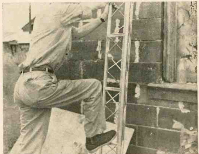
Fig. 1, left—Fringe-area antennas mounted on tower. Horizontal boom is made of mast section and supports the right side of tower where no guy wires could be erected Fig. 2, right—Tower steps permit climbing, facilitating adjustments, replacements or repairs.
