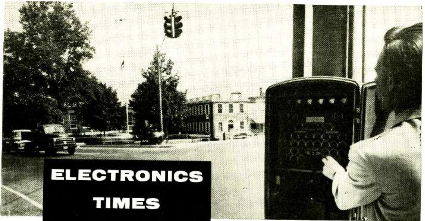
Technician adjusts timing on traffic signal.
