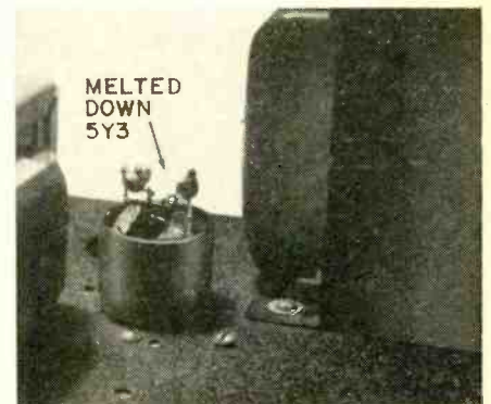
Fig. 5—The guilty 5Y3, with glass removed to show the melted parts.
