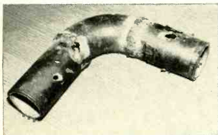
Enemy attack. This section of gas main was holed in three places by galvanic corrosion.
