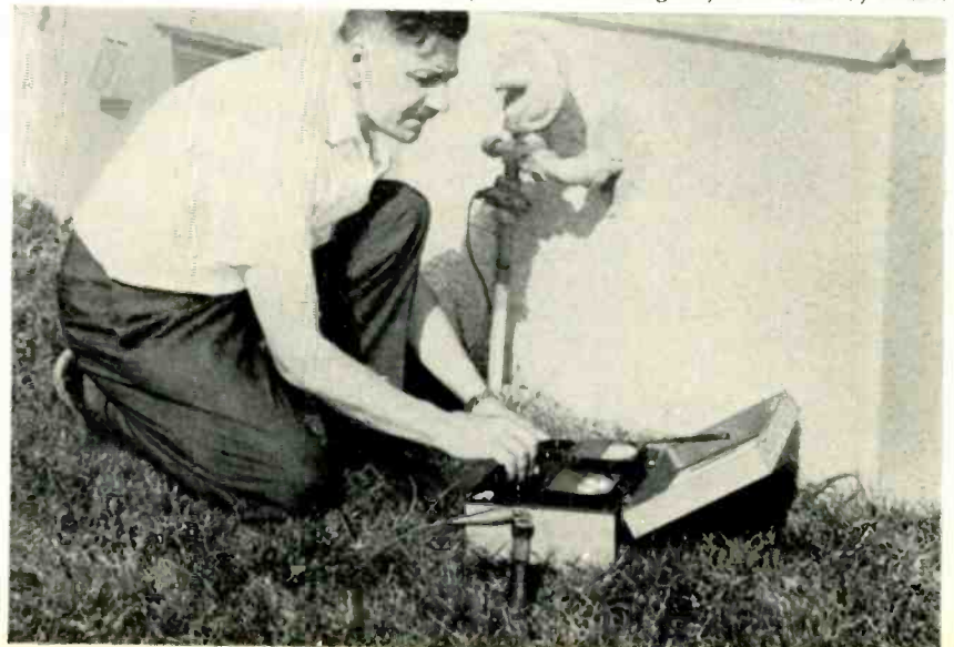
Using a special-purpose multimeter to check the cathodic protection voltage of a section of main.
