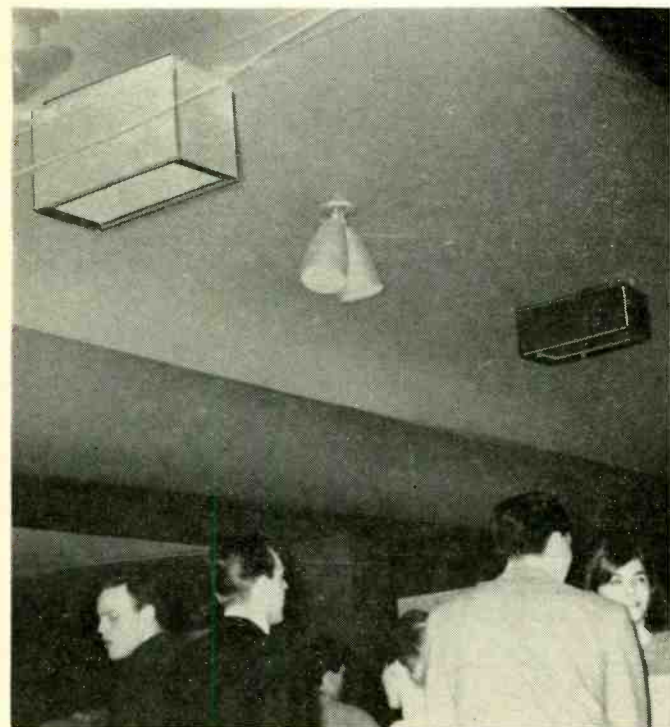
Sealed hi-fi enclosures on the ceiling are the mainstay of the dance-floor sound distribution.
