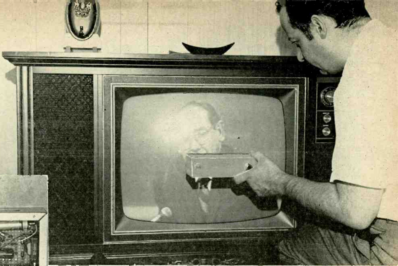
CHECK THE FACEPLATE for x-rays too. Scan the entire front of the screen slowly. At left is a closeup of the detector. This set had no x-ray problem.
