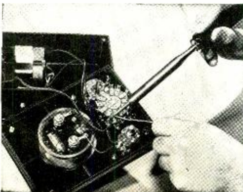
Construction of Multimeter.
