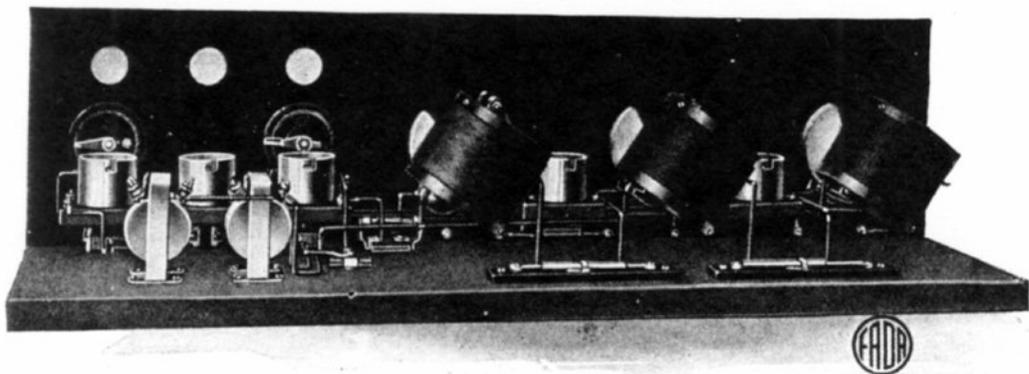
Showing the rear view of a five-tube Neutrodyne circuit radio receiver constructed according to information in the booklet "How to Build Hazeltine Neutrodyne Circuit Radio Receivers."
