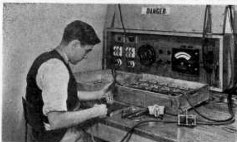
Fig. 3. Completed condensers are carried in trays to the testing bench where, thru heavily insulated electrodes, 1,000 volts is applied to the terminals.
