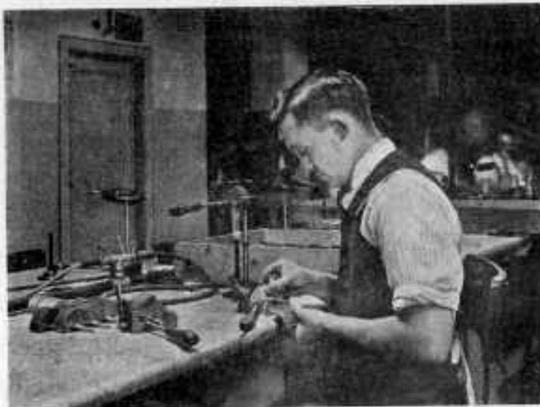
Fig. 2. The operator is assembling plates in one jig, another is being heated, while a third is cooling on the bench. Thus the soldering operations continue without delay.
