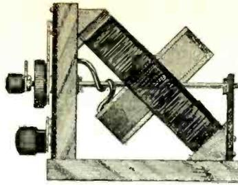
Fig. 30. Rotary receiving tuner, or vario-coupler, of 1913. Both primary and secondary coils are tapped. The inside, secondary, coil is rotated by the knurled knob on the shaft.
