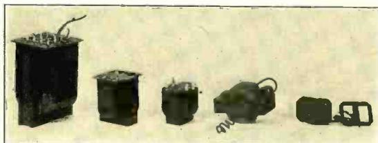
A few radio transformers, choke coils and punchings made of electrical sheets.
