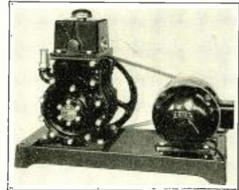
pump. At a speed of 425 r.p.m. it reaches a pressure of one micron in one fifth of the time required by the Cenco Megavac pump.
