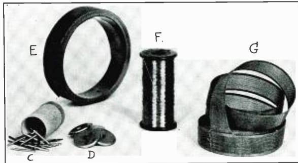
C. Cathodes for type 27 tube made from "Svea" plate.
