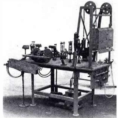
bination cutting, welding and trimming machine upon which flexible cable may be cut apart or two pieces joined and trimmed without unraveling and at the same time maintain practically the same flexibility as it had before.
