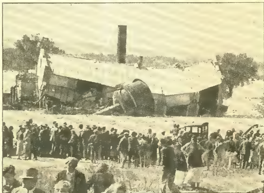
The crowds in McCook as they watched the building housing the power plant topple into the flood waters
