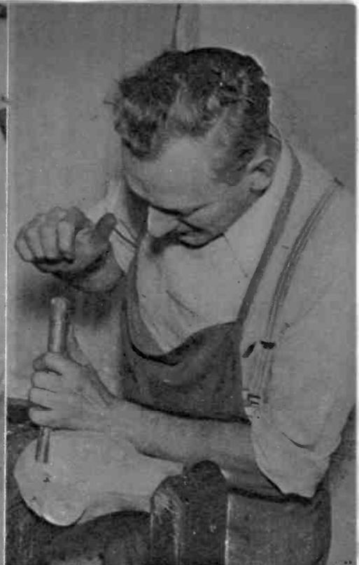
7 The next step is to hollow out both halves of the head. Again Frank uses the hand chisel
